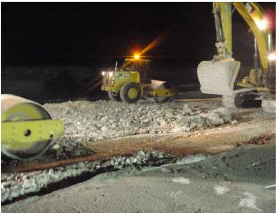
Photo 12: Two vibratory packers and 330 Excavator placing ROQ material around 1+40
