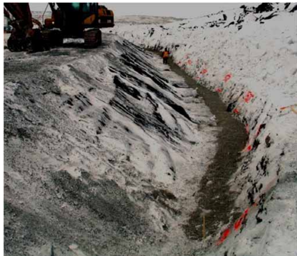
Photo 8: Bentonite over liner Sta 5+85 facing west (to Sta 5+30)
