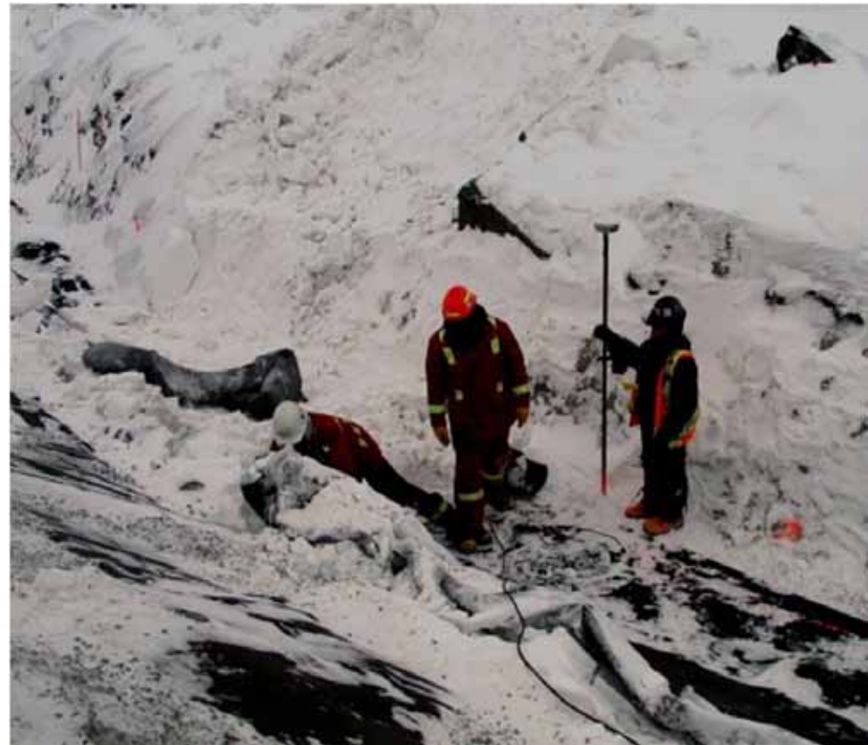
Photo 11: Layfield repairing HDPE liner at Sta 5+24
