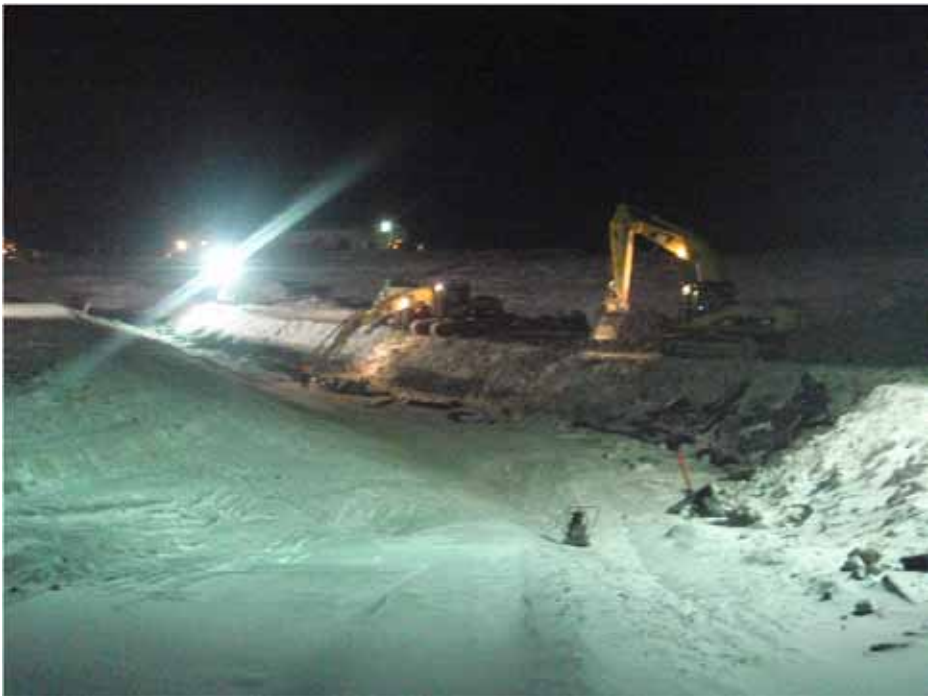
Photo 16: ~NEN view of excavators working on removing the protective HDPE liner over the fillet GCL.
