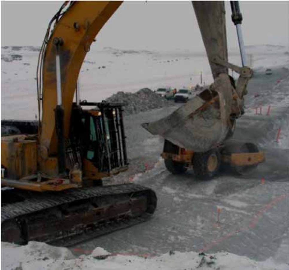
Photo 2: Placing FCM at the south end.
