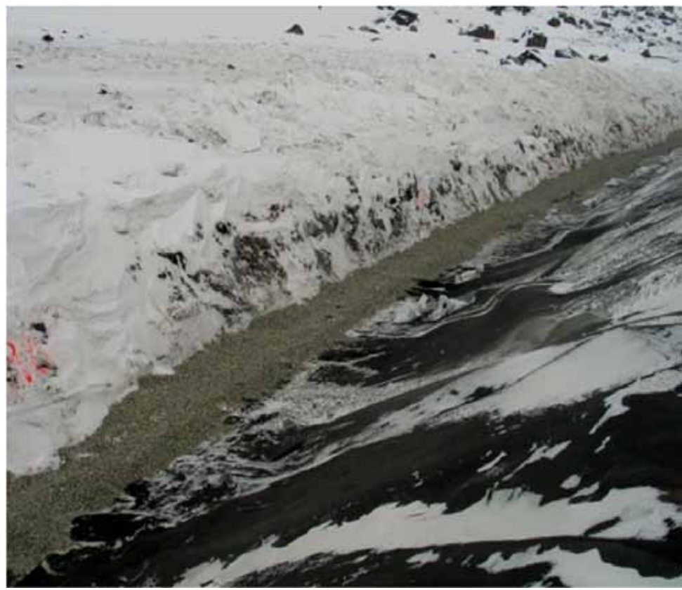
Photo 9: Bentonite over liner Sta 3+85, facing east (to Sta 4+45)
