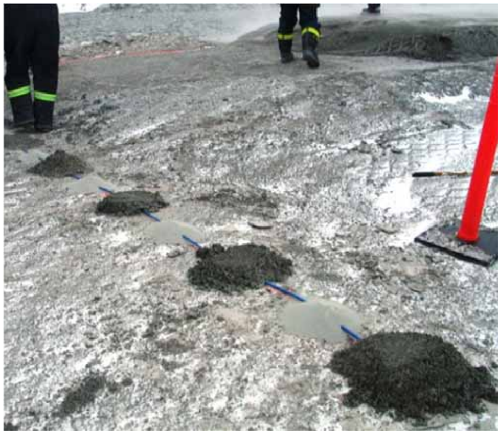
Photo 6: Installation of multi bead thermister ND- HTS-040-33.5
