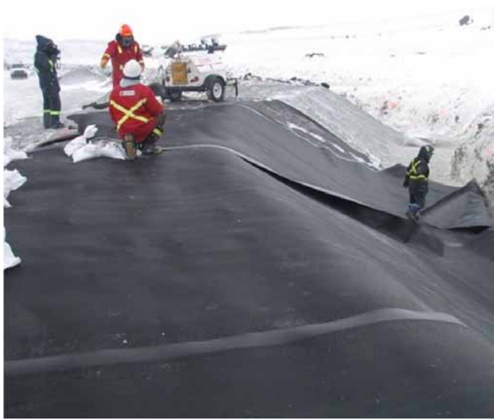
Photo 10: Layfield placing HDPE between Sta. 3+35 and Sta 3+85
