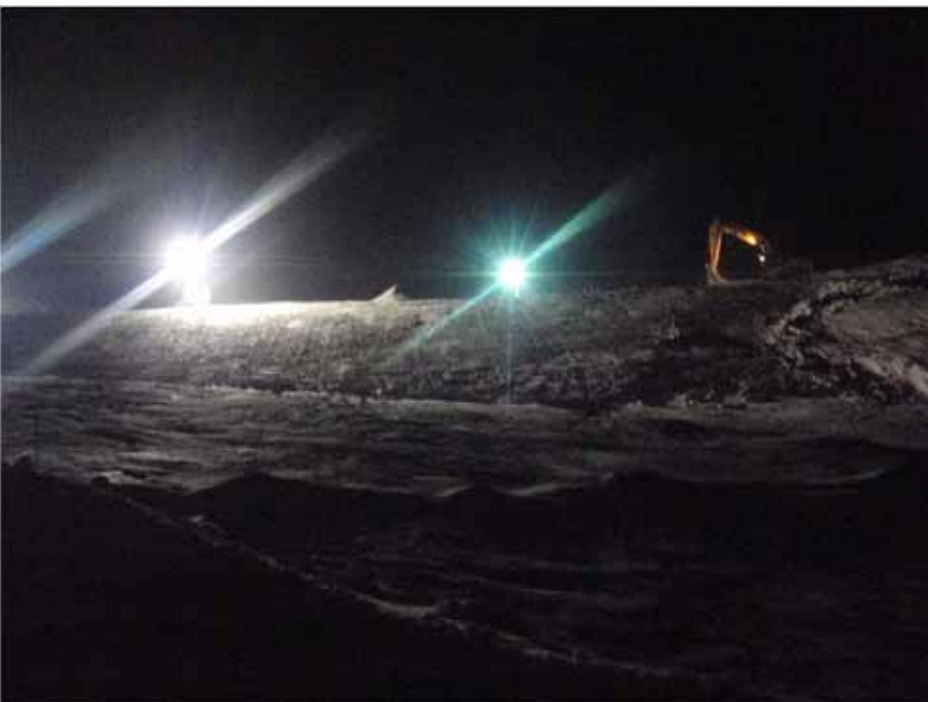
Photo 15: ~SE view of downstream dam shell after 4H:1V sloping.
