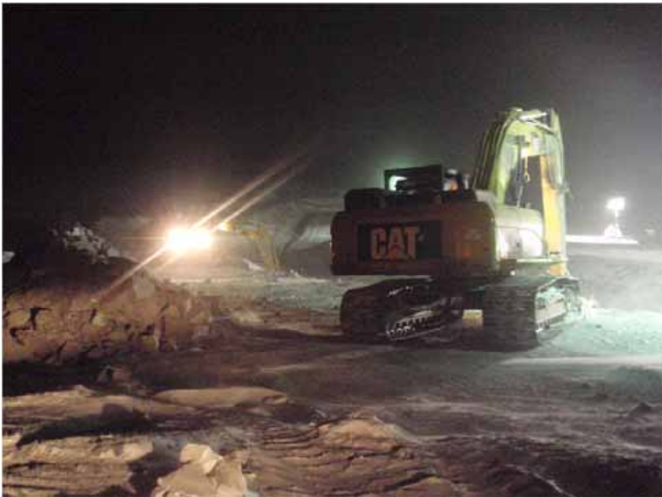
Photo 17: ~WSW view of excavators working on removing HDPE liner and pulling back ROQ on upstream slope.
